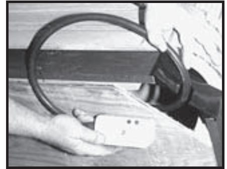
Ground fault interrupter plug & power cord fished through arched corner of the spa
