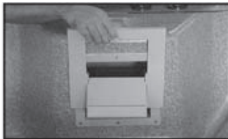
2. Remove Front Filter Plate
